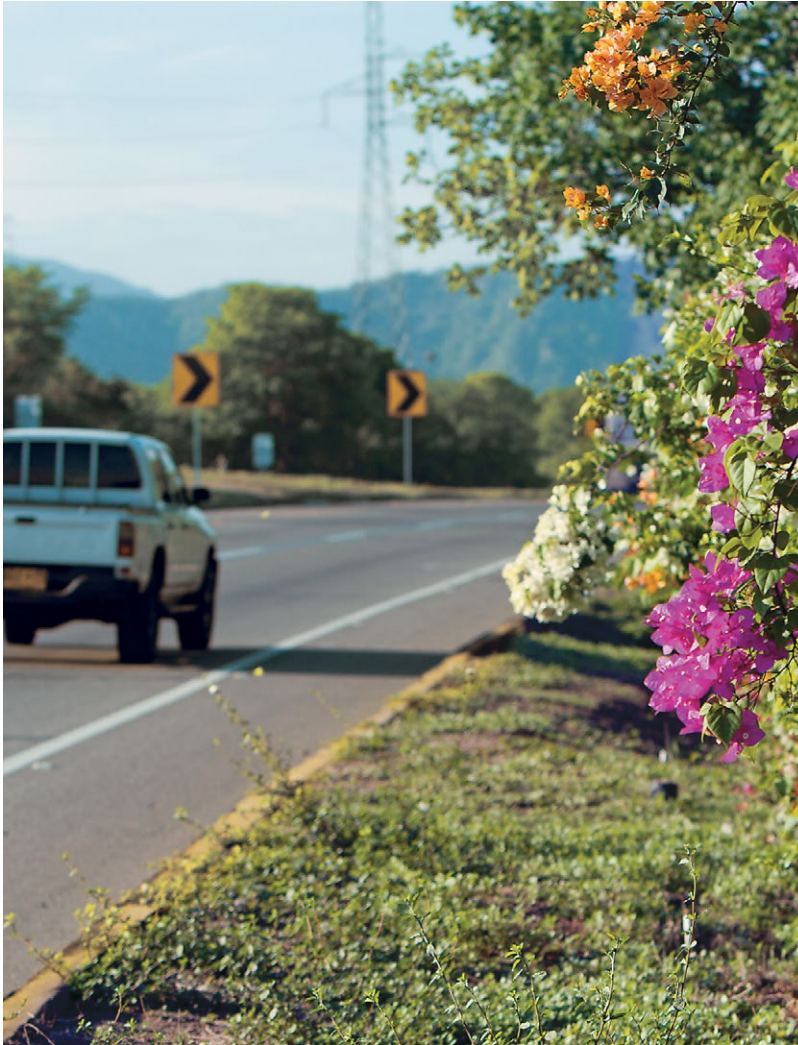
↑ The Coal Road paved.
